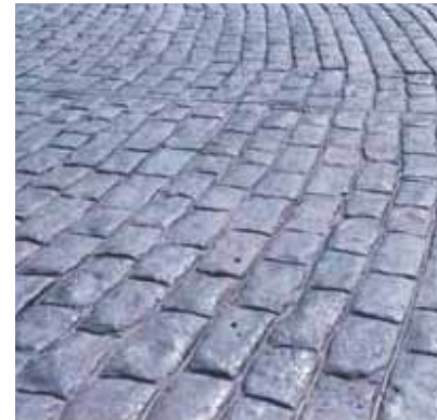
STAMPED, COLORED CONCRETE will act as a rumble strip outside of crosswalks
