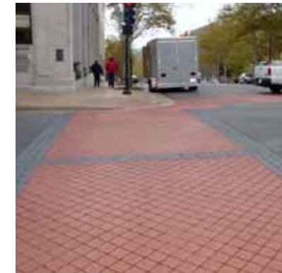
CROSSWALKS use stamped concrete to provide contrast and longevity
