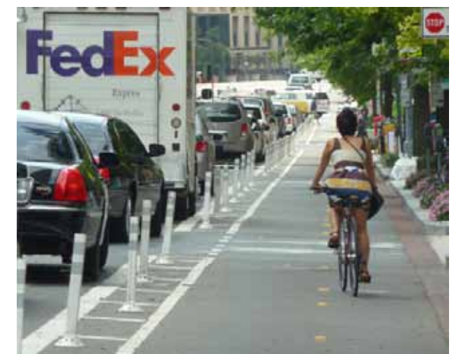
A cycle track is more protective than a standard bike lane, so it can accommodate multiple levels of cyclists. A safety buffer separates its parallel inbound and outbound lanes from on-coming traffic or parked cars.
